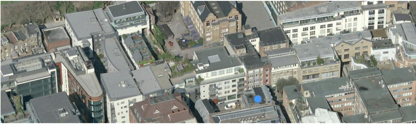
Image 1: Aerial view of street elevation
